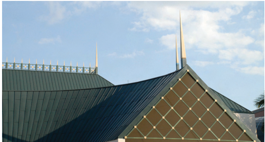
Naples Philharmonic, Naples, FL (completed; SOLARGARD® 6083 and SOLARGARD® Acrythane)
